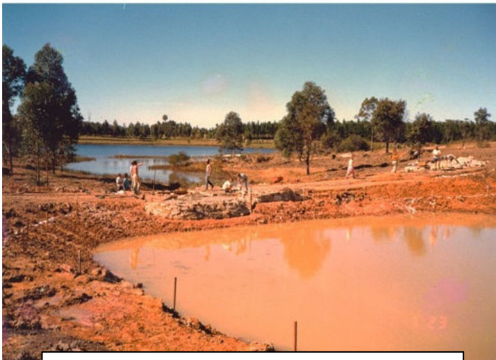
The lagoon at Noosa Botanic Gardens under construction.
